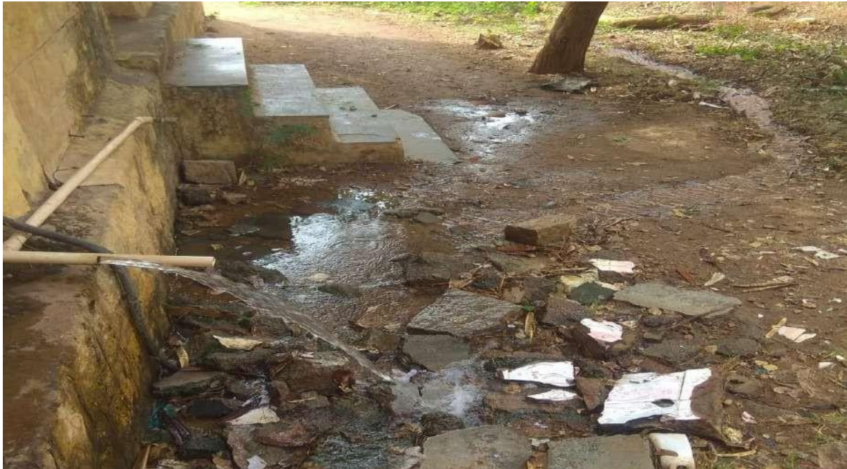
Waste water generated through R.O. plant is channelized to plantations
